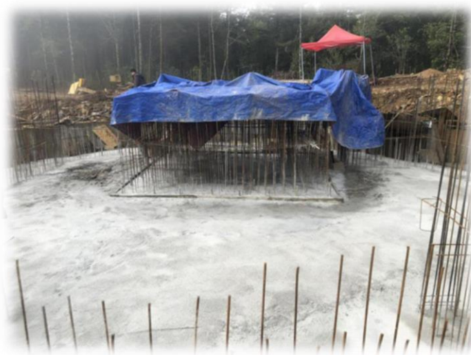
图 3.5：基墩和建筑物基础浇筑(1.5 米以下) Concreting the telescope base pier trough and the foundation of the telescope main building (up to -1.5m of the ground level)
