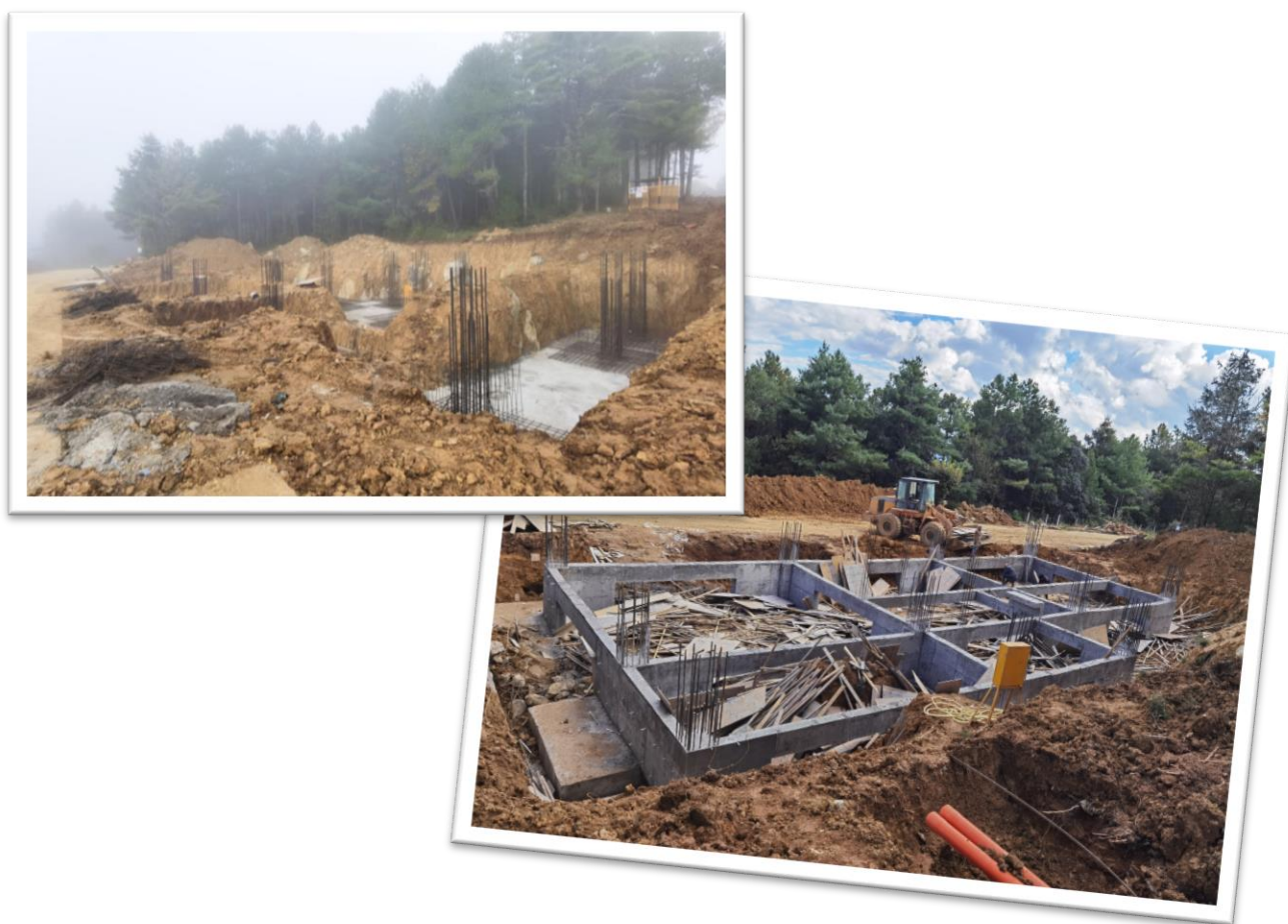
图 3.11: 左: 数据中心基础钢筋绑扎; 右: 数据中心完成基础浇筑 Left: foundation reinforcement binding of the data center; right: foundation pouring of the data center completed
