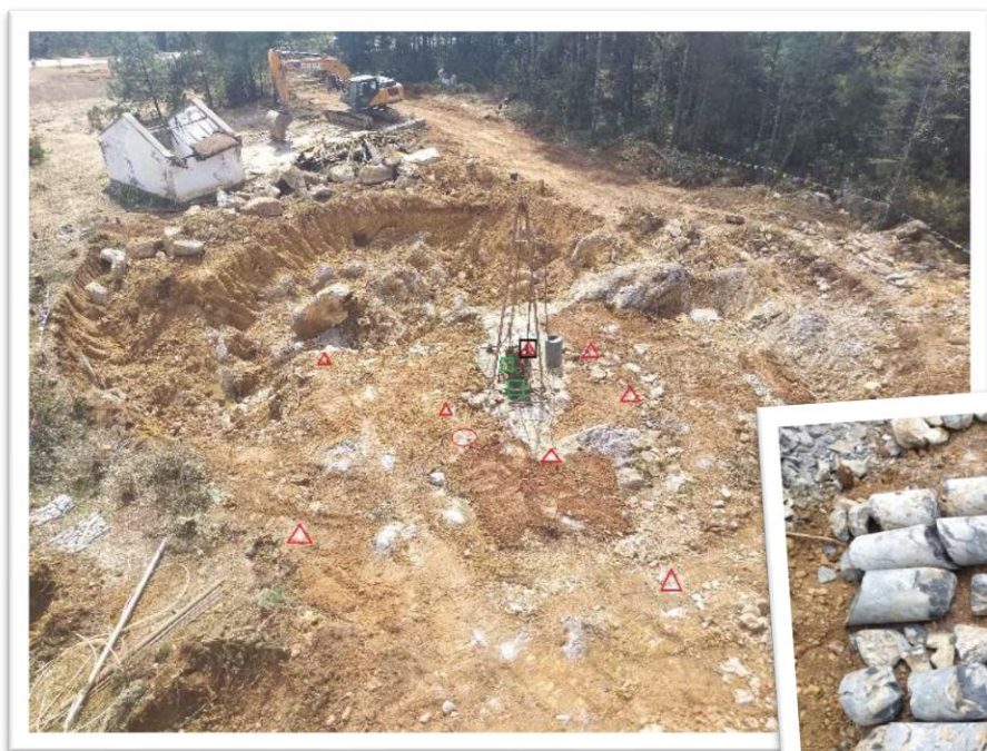
图 3.4：地勘钻孔位置分布 Geological drilling for the telescope main building
